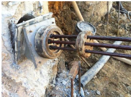
Load Cells (Hydraulic, Strain Gauge or Vibrating Wire)
