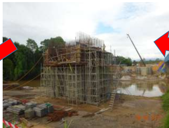
Hammerhead (Bottom Slab)
