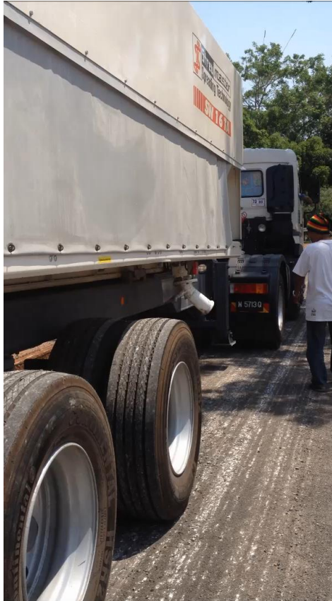
Track record 3 : Spreading cement.
