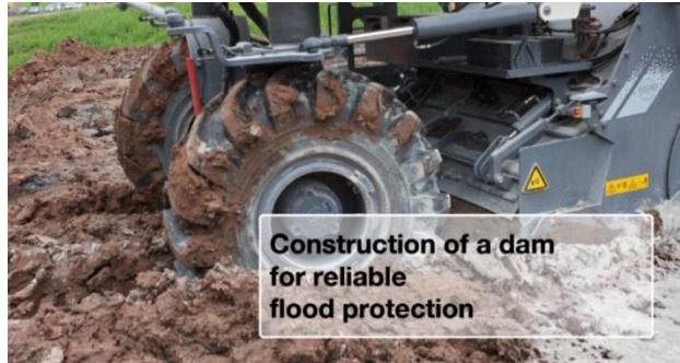
Soil stabilization at peat area
