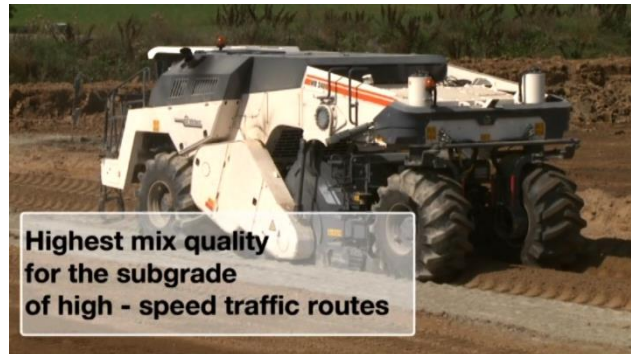
Soil stabilization at subgrade level for highway
